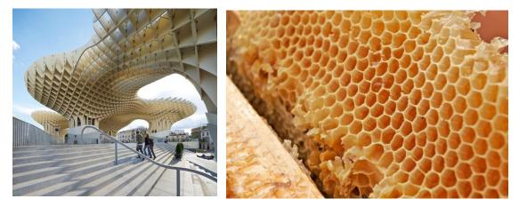
The structure of Metropol Parasol at Seville was inspired from the honeycomb for achieving such large spans between the columns.
