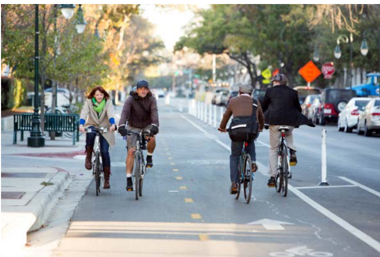
Main vehicular roads in Portland segregated into further smaller bicycle ways and broad sidewalk along with landscape to facilitate sustainable commute.
